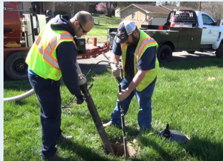
We will be using hydro excavating
